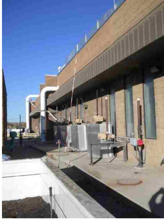
Figure 27 South Side of PTF - Looking Downstream Along Effluent Channel
